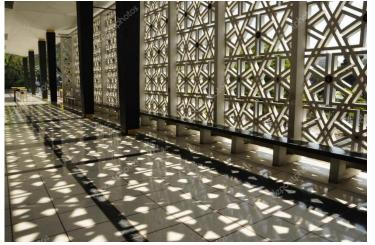
Figure 11 Concrete wall façade
