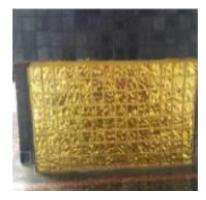
Figure 7 Laminated golden aluminum mosaic tiles on columns design
