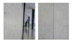
Figure 8 Reinforced concrete walls covered with Italian marble
